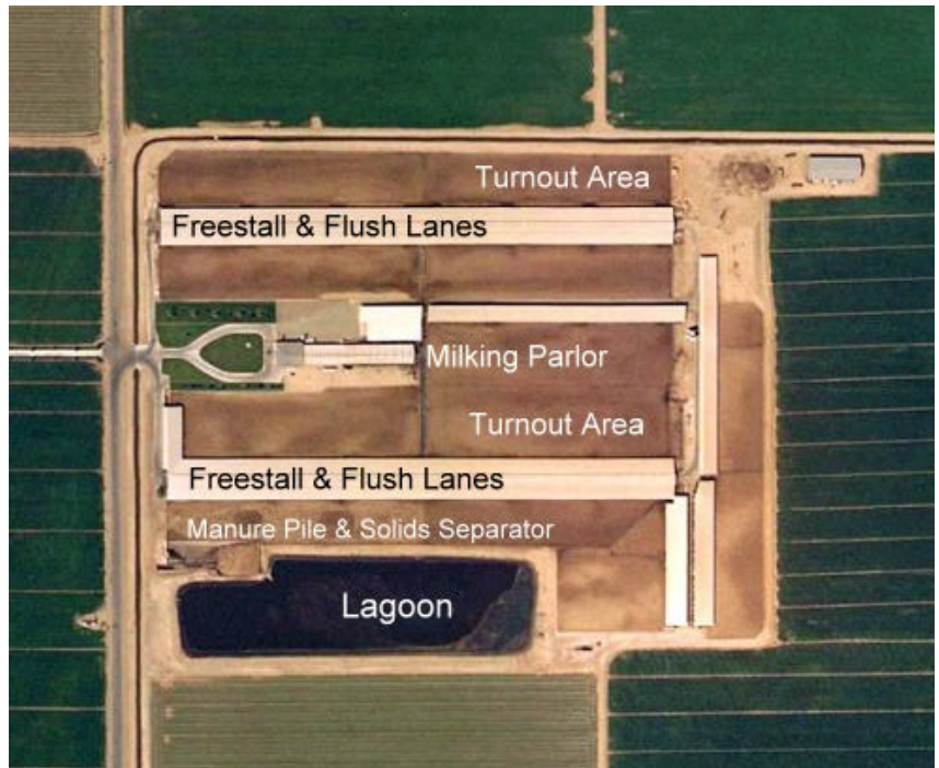
Figure 3. Aerial Photo of a Freestall Flush Lane Dairy.
