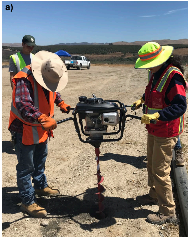
Figure 3.13 Installation of Thermocouple Array and Field Temperature Measurement
