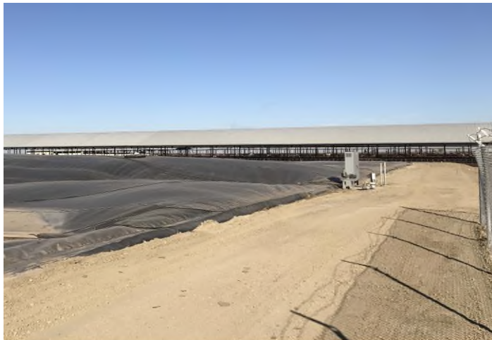
Covered dairy digester lagoon
